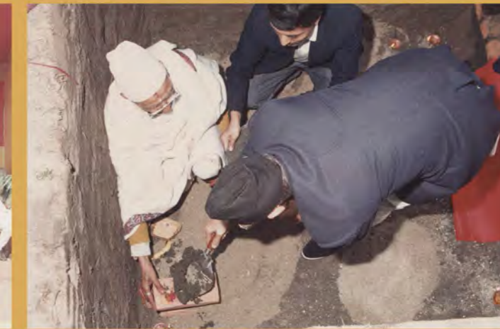
The then Rt. Honorable Prime Minister GP Koirala laying the foundation stone of the FNCCI building, 1995
